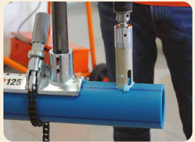
2 - Accurate centering of drilling area
